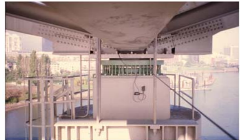
Figure 13 - Isolator with double tapered pin steel hysteresis dissipating element used for the seismic retrofit of the Marquam Bridge, Oregon, USA.
